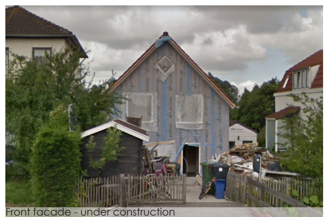
Front facade - under construction
